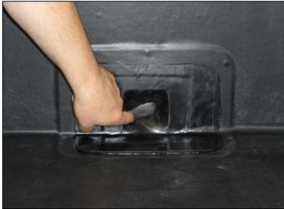
2) Install Uncured PS tape to the outlet. This should be large enough to join onto the membrane by a minimum of 50mm. Cut a small square out of the middle of the tape and mould the tape into the outlet pipe by 25mm. Cut a second section of Uncured PS tape 100mm wide. This will be inserted into the outlet pipe to reinforce and lengthen the tape that was turned into the pipe by 25mm. Apply ClassicBond Primer to outlet pipe and to already installed tape before application.
