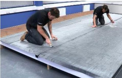
3) Lay the top membrane onto the Seam Tape. Pull away the poly backing from the tape at a 45° degree angle to the seam. While removing the poly backing, draw your hand across the seam, from the back to the leading edge. Roll the seam at right angles to the seam direction, not along it.
