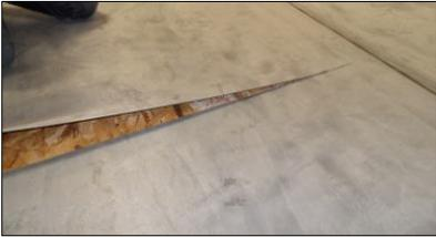
1) Ensure there is no gap between the membrane when butt jointing. The 150mm tape should be centrally located over the joint.
