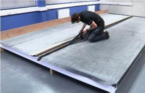
2) Using moderate pressure set the Seam Tape into place to keep air from being trapped under the tape and unroll the 75mm wide tape along the length of the seam, aligning the Seam Tape (not the clear backing) along the chalk line. Care must be taken not to get any bubbles or wrinkles in the tape.
