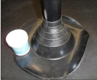
1) Cut the ClassicBond PS Pipe Seal above the raised "rib" one size smaller than the pipe diameter. DO NOT CUT THROUGH THE RIB. Pull pipe seal over pipe until base flange is in contact with the ClassicBond EPDM membrane.
