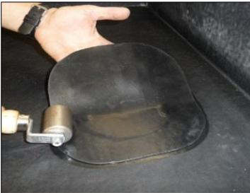
2) Apply the Uncured PS tape to the primed area. Once fitted cut a small section from the centre of the tape out to expose the outlet opening and press the remaining tape down into the outlet. Roll the entire flashing with hand roller.
