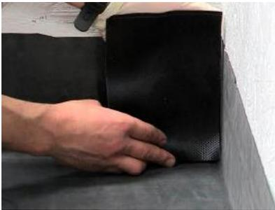
2) Cut an appropriate size piece of 225mm uncured flashing (min. 50mm wider than the flap of membrane), press the flap back to the upstand and install the uncured flashing tape.
