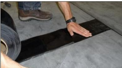
3) Once the ClassicBond Primer has dried, peel back 150mm of the poly backing and press the PS tape into the primed area. Once the tape is held in position, peel back the poly backing and smooth the tape into the primed area. Progress along the seam.
