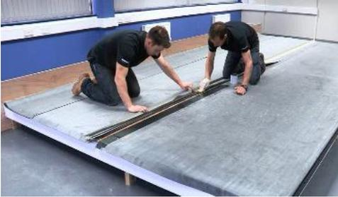
1) Fold the top sheet back to expose the seam area. Using a scrubbing pad apply the ClassicBond Primer to the seam area. Apply the primer past the seam edge to the line. ClassicBond Primer must be dry before application of PS tapes.
