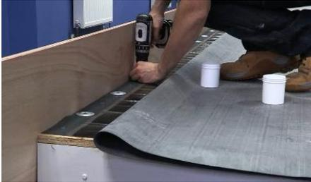
1) Mechanically fasten the RUSS horizontally into the decking or into the upstand with the PS section being to the inside of the roof.
