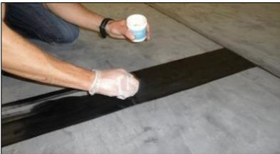
2) Apply ClassicBond Primer to the area to be seamed. Apply primer 80-100mm either side of the join in the EPDM sheets.
