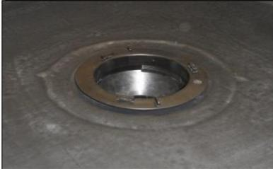
3) Insert a bead of ClassicBond Water Cut Off mastic between the underside of the membrane and the top flange on the outlet. Screw in the clamping ring till it's completely tightened. Use the two tightening lugs to apply leverage to the ring.
