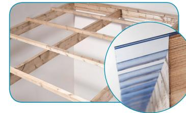
Sheets should overhang the roof by 60mm to allow rainfall to run-off into the gutter and should be wide enough to cover the barge board at the side.
