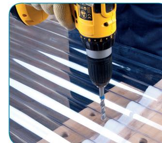
Drill sheets singly with a masonry bit, using a low speed drill and light pressure. Support the sheet securely under each hole position when drilling.
