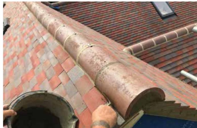
Above: A mechanically fixed mortar bedded ridge
