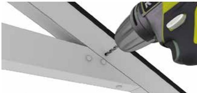
**3** Using a 6mm bit, drill a hole through the rafter and tie bar brackets.
